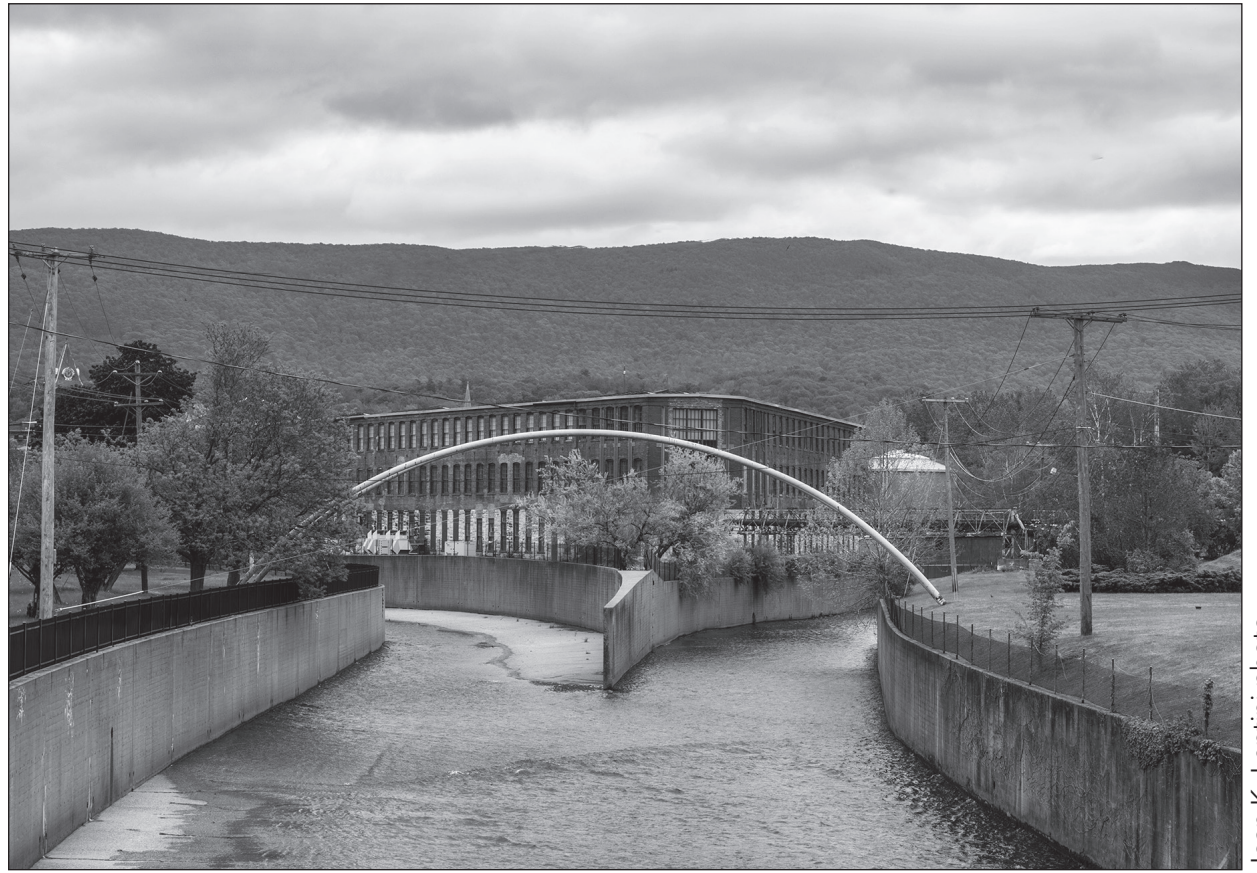
Seen from the Brown Street bridge, the north and south branches of the Hoosic River converge just west of downtown North Adams, each contained within massive concrete chutes built in the 1950s.
